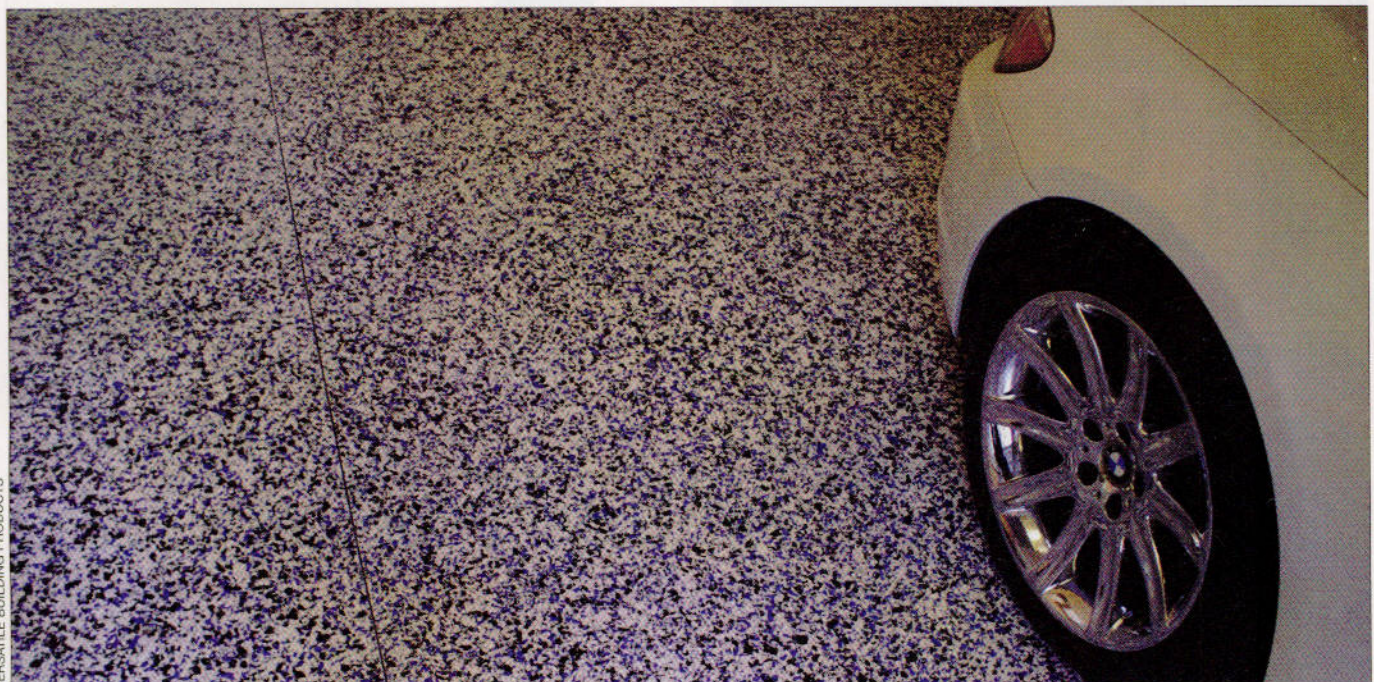
It took only four hours for two men to coat this concrete garage floor.
